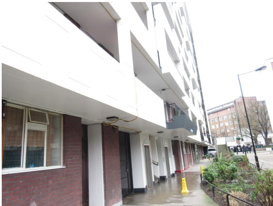
Close up of access decks
