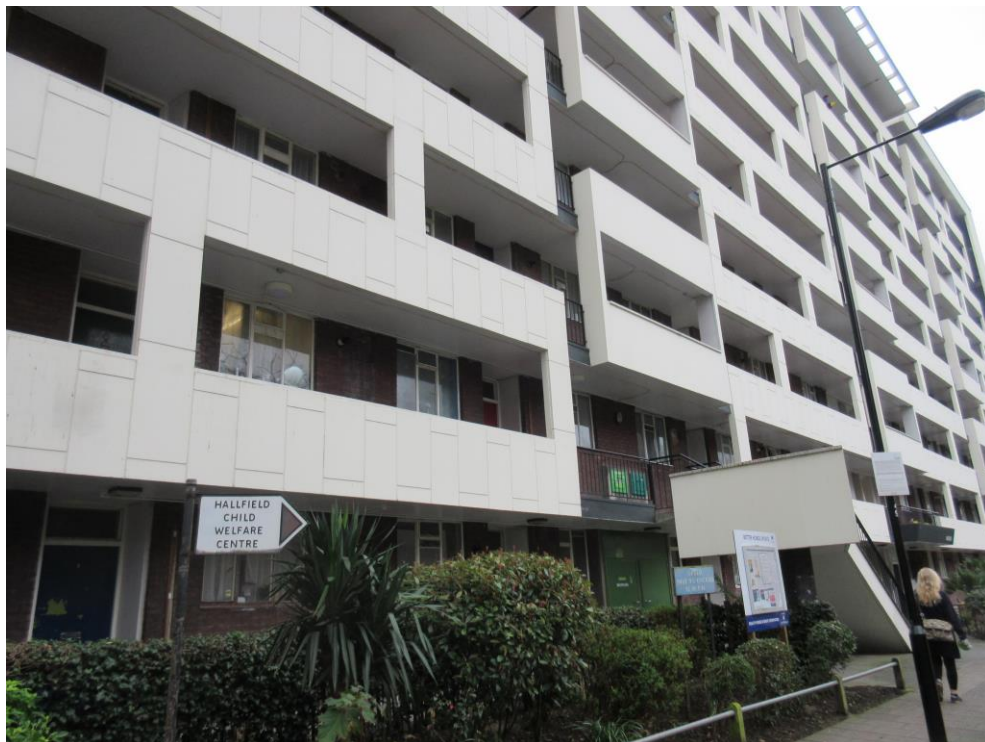
North elevation showing walkways
